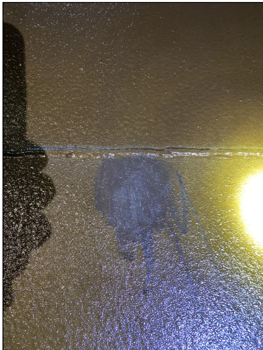
Photo 31 – Tank floor coating
