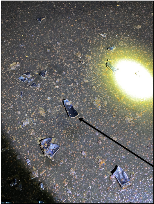
Photo 13 – Tank floor and failed coating flakes from roof rafters
