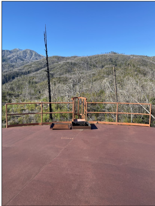
Photo 7 – Exterior ladder and guardrail at tank roof
