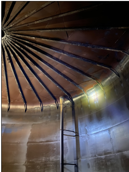
Photo 35 – Roof rafters at knuckle and overflow pipe
