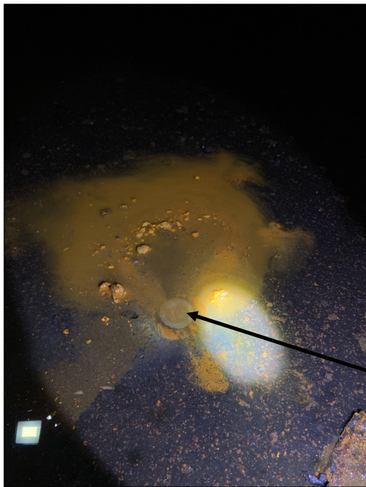
Photo 11 – Tank floor corrosion pit
