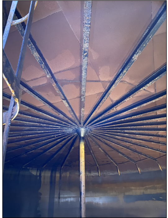
Photo 46 – Center column viewed from interior ladder
