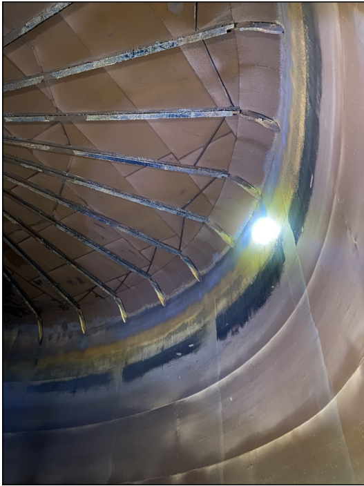
Photo 33 – Roof rafters at knuckle
