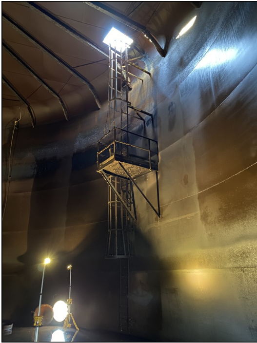
Photo 37 – Interior tank ladder
