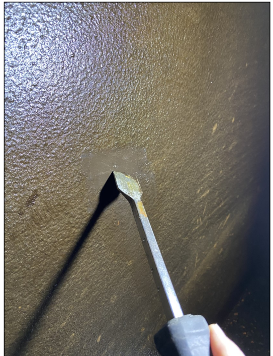
Photo 36 – Tank wall coating
