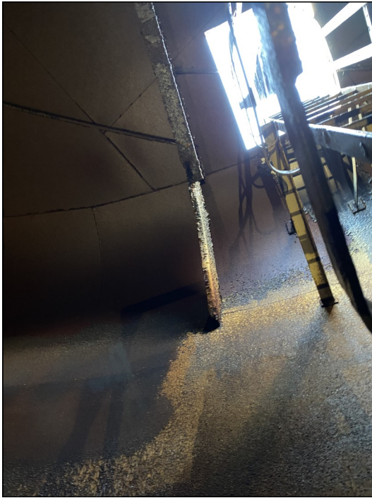
Photo 45 – Looking up at the roof hatch and interior tank ladder
