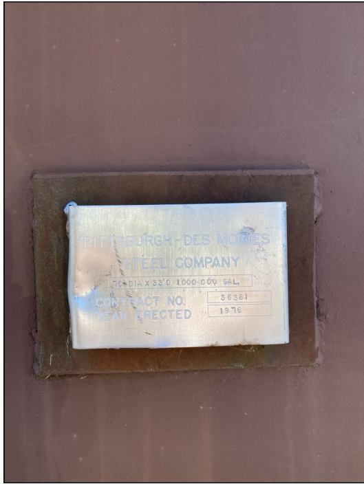
Photo 1 – Tank nameplate: Pittsburgh-Des Moines Steel Company; 70' DIA X 33'; 1,000,000 GAL; Contract No. 36381; Year Erected: 1976
